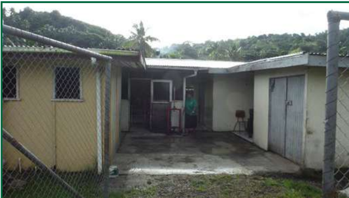
Figure 15: Small Scale Processing Facility, Rabi Island, Fiji
