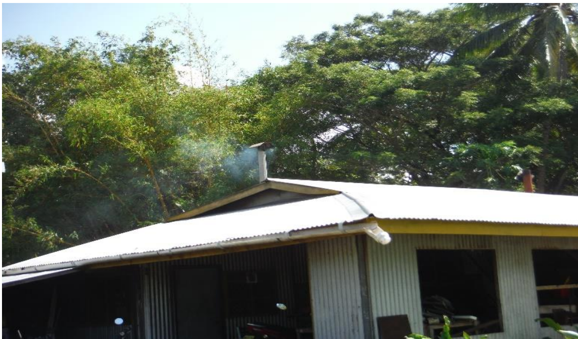
Figure 1 Well sited copra mill. The smoke is removed efficiently by the prevailing wind
