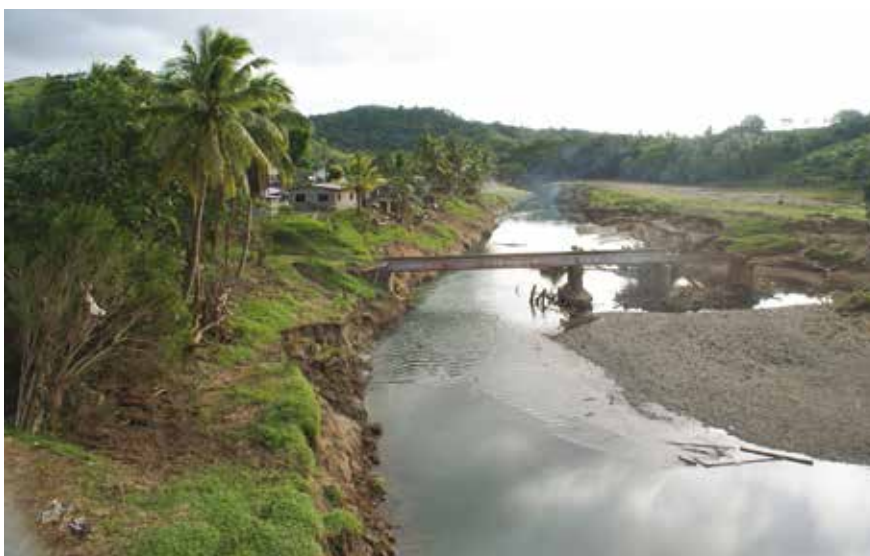
Infrastructure damage from cyclone Evan, Samoa
