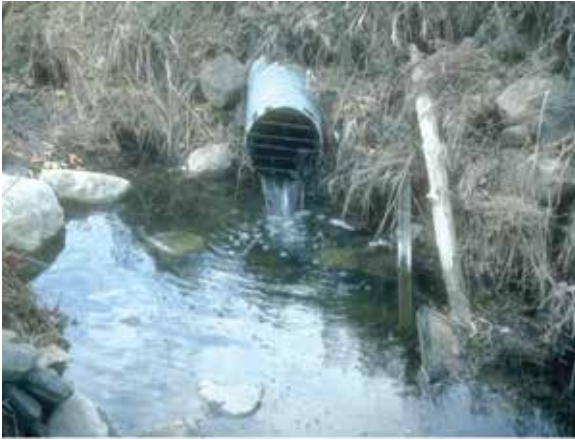
Figure 17.19. Subsurface drain line discharges into an edge-of-field ditch, diverting groundwater to surface waters.
