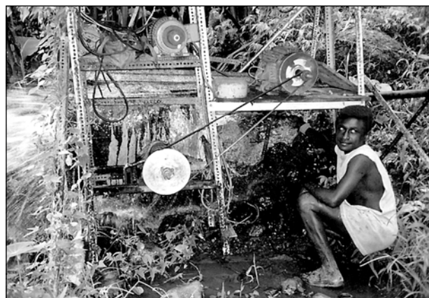
Picohydro electricity, like this unit in Bougainville, holds potential as an energy source for remote villages.
