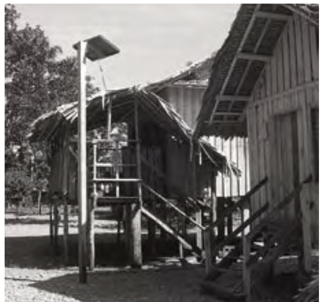
Battery charging enterprise — a photovoltaic panel supplies electricity to charge batteries (see energy report opposite).
